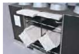
Removing filters and Lossnay recovery module
